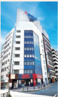
Akasaka-Mitsuke Station Front I Formed in March 2026 Total amount of funding: ¥2.00 billion
